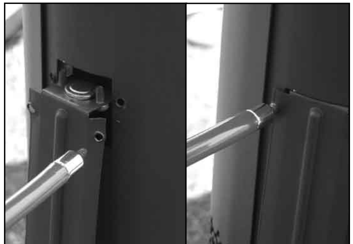
Figure 27: Spill switch installation.
